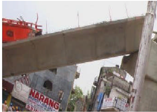
METRO RAIL BRIDGE, INDIA
