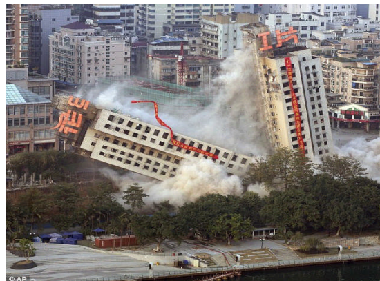
APARTMENT BUILDING SPLITS INTO TWO, FALLS SIDEWISE
