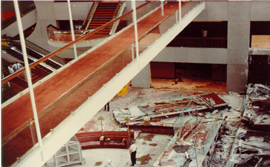
HYATT REGENCY WALKWAY COLLAPSE
