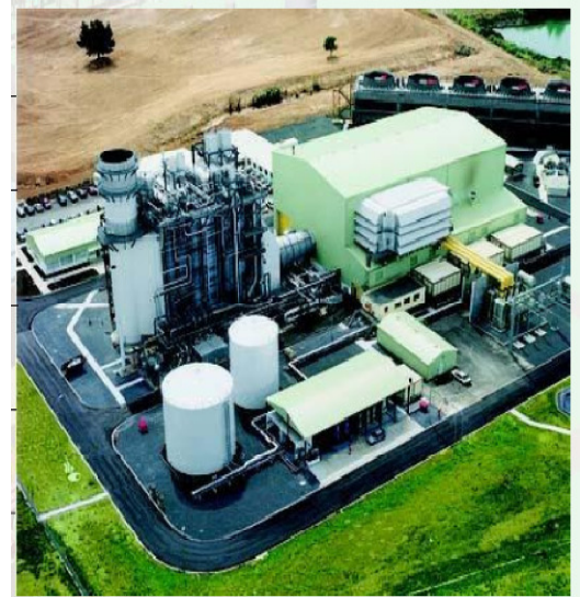
POWER PLANT PROJECT
